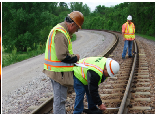
Examining the railway near a nuclear power plant
