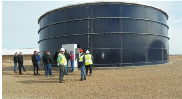
Millan (red hard hat) at the firewater pump and tank design build request for proposal pre-bid site walk.
